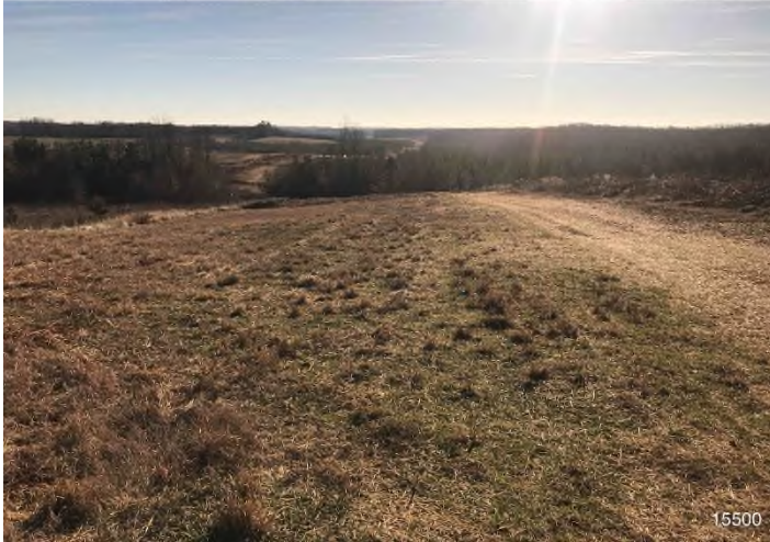
Figure 1: STA 15500+00 – Controls in place and functioning properly. Area stabilized with straw. BRG: 123°SE (T) LAT: 36.906035 LON: -79.474116 ±32ft ALT: 952ft
