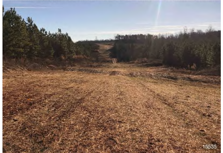
Figure 2: STA 15535+00 – Controls in place and functioning properly. Area stabilized with straw. BRG: 95°E (T) LAT: 36.900461 LON: -79.464243 ±16ft ALT: 832ft
