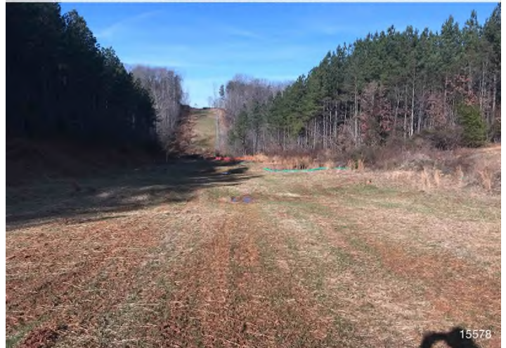
Figure 4: STA 15578+00 – Controls in place and functioning properly. Area stabilized with straw. BRG: 307°NW (T) LAT: 36.892059 LON: -79.439800 ±21738ft ALT: 756ft
