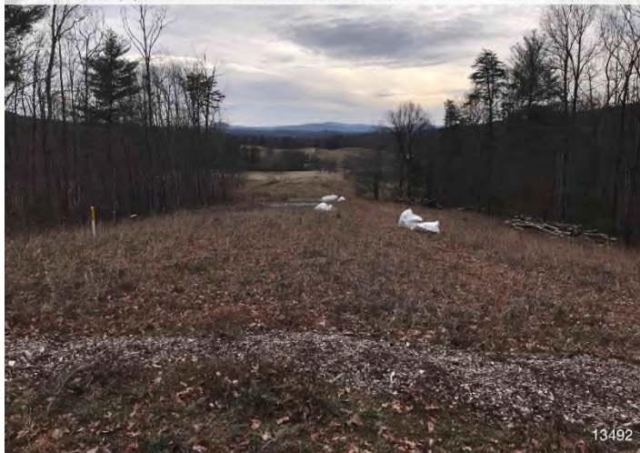
Figure 3: STA 13292+00 – Controls in place and functioning properly. BRG: 160°S (T) LAT: 37.114868 LON: -80.056258 ±16420ft ALT: 1859ft
