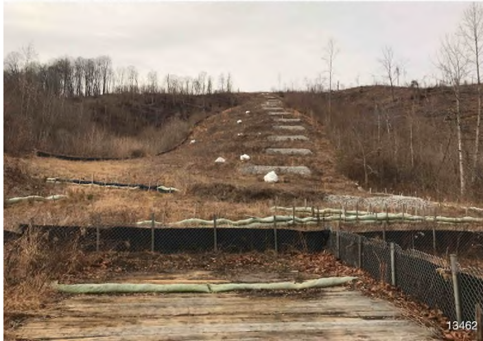
Figure 1: STA 13262+00 – Controls in place and functioning properly. BRG: 320°NW (T) LAT: 37.115549 LON: -80.060545 ±32ft ALT: 1459ft
