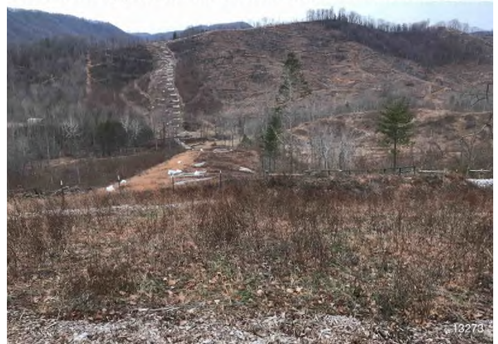
Figure 2: STA 13273+00 – Controls in place and functioning properly. BRG: 294°NW (T) LAT: 37.115486 LON: -80.056203 ±32ft ALT: 1644ft
