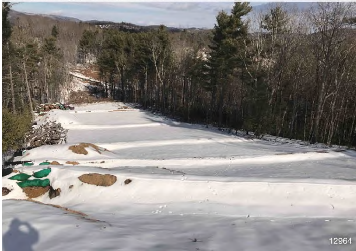
Figure 3: STA 12964+00 – Controls in place and functioning properly. BRG: 13°N (T) LAT: 37.132743 LON: -80.137531 ±98ft ALT: 2653ft
