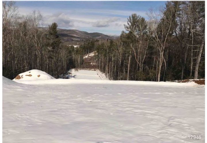
Figure 4: STA 12946+00 – Controls in place and functioning properly. BRG: 353°N (T) LAT: 37.136174 LON: -80.138652 ±32ft ALT: 2718ft
