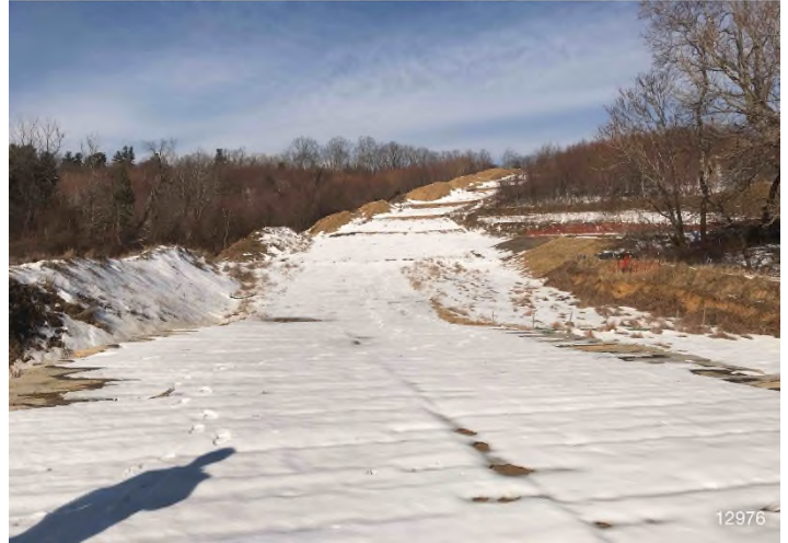
Figure 2: STA 12976+00 – Controls in place and functioning properly. BRG: 314°NW (T) LAT: 37.130091 LON: -80.136250 ±98ft ALT: 2693ft
