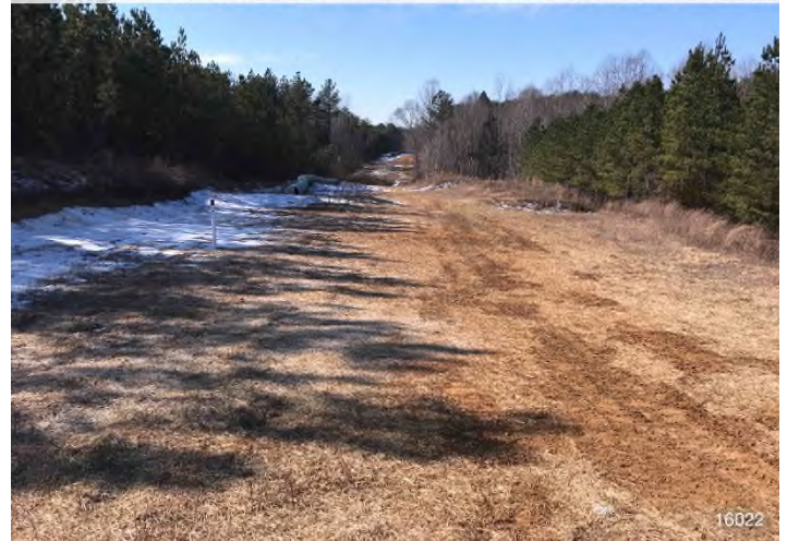
Figure 4: STA 16022+00 – Controls in place and functioning properly. Area stabilized with straw.
