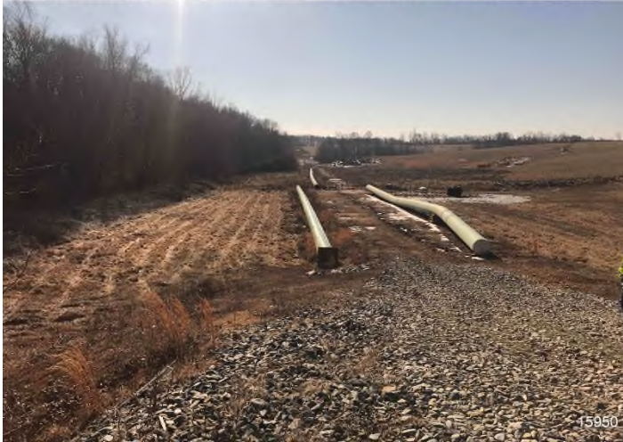
Figure 3: STA 15981+00 – Controls in place and functioning properly. Area stabilized with straw.
