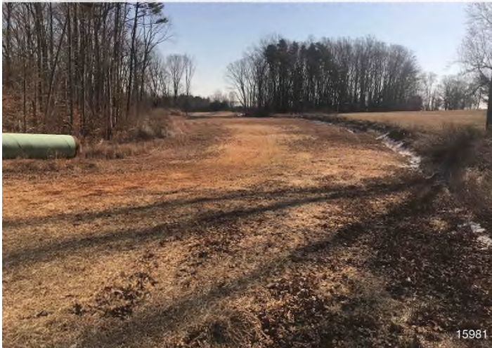
Figure 3: STA 15981+00 – Controls in place and functioning properly. Area stabilized with straw.
