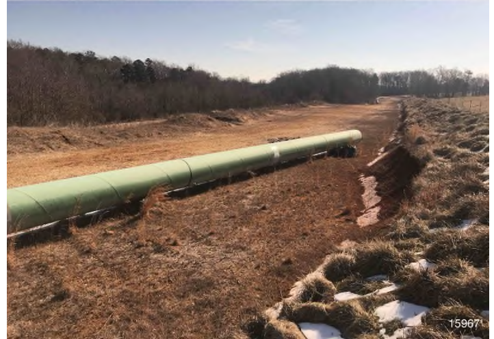
Figure 4: STA 16022+00 – Controls in place and functioning properly. Area stabilized with straw.
