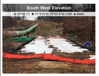
Figure 3: ESC's are in place at designated crossing S-KL38.
