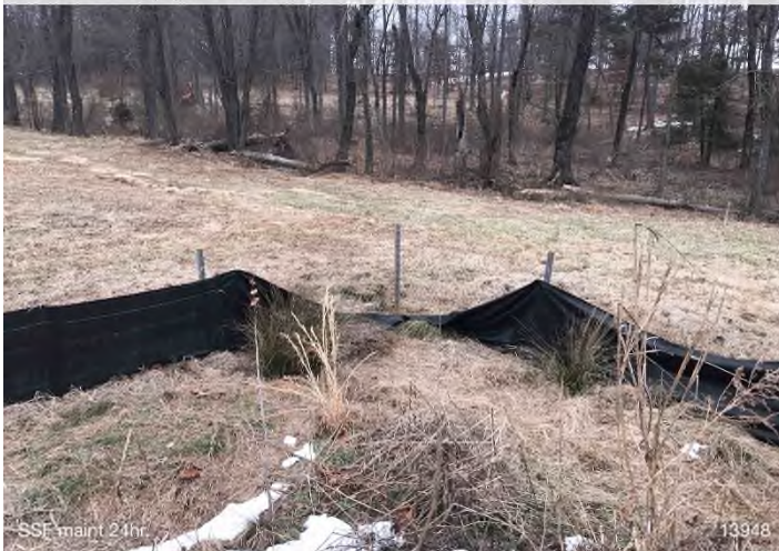
Figure 3: STA 13948+00 – SSF repair needed. BRG: 50°NE (T) LAT: 37.047815 LON: -79.898022 ±98ft ALT: 1042ft
