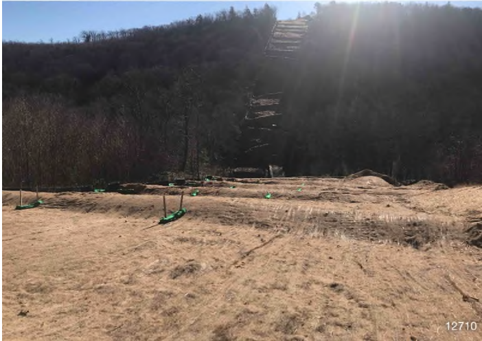
Figure 3: STA 12710+00 – Controls in place and functioning properly. Area stabilized with erosion matting. BRG: 144°SE (T) LAT: 37.188799 LON: -80.151953 ±164ft ALT: 2997ft
