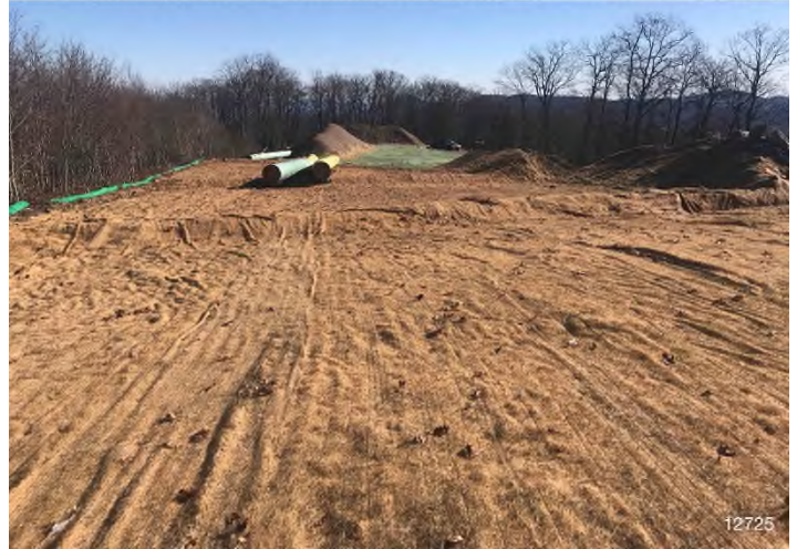
Figure 2: STA 12725+00 – Controls in place and functioning properly. Area stabilized with erosion matting. BRG: 114°SE (T) LAT: 37.185484 LON: -80.149804 ±16ft ALT: 3397ft
