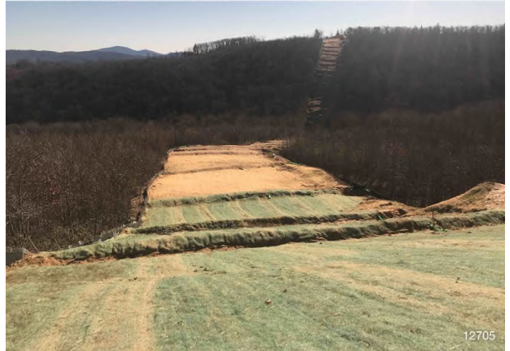
Figure 4: STA 12705+00 – Controls in place and functioning properly. Area stabilized with erosion matting. BRG: 149°SE (T) LAT: 37.190526 LON: -80.153287 ±164ft ALT: 3341ft
