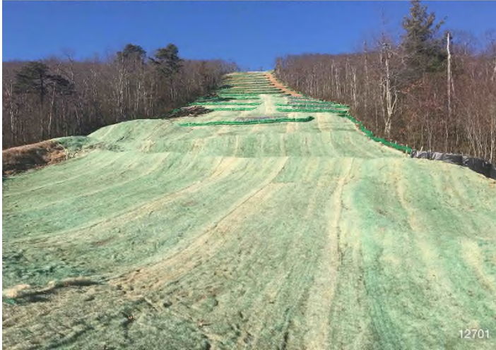
Figure 1: STA 12701+00 – Controls in place and functioning properly. Area stabilized with erosion matting. BRG: 302°NW (T) LAT: 37.190745 LON: -80.153811 ±16ft ALT: 3353ft
