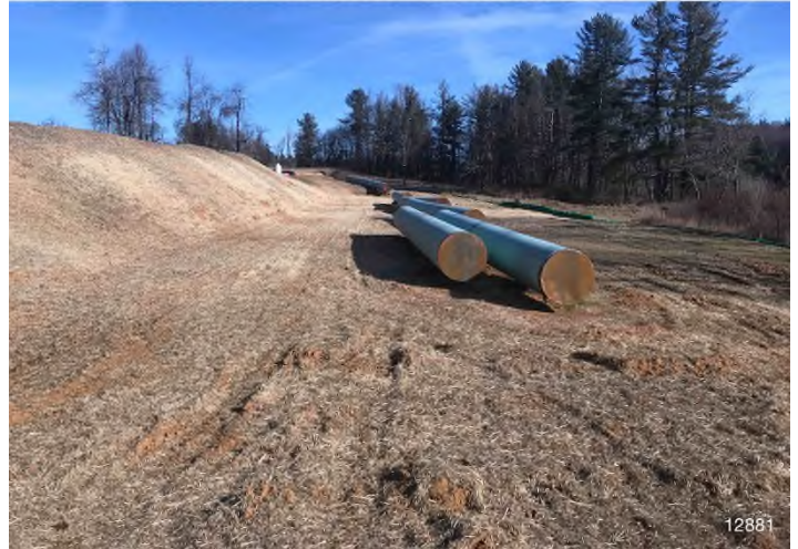
Figure 4: STA 12881+00 – Controls in place and functioning properly. Area stabilized with straw. BRG: 45°NE (T) LAT: 37.148881 LON: -80.119800 ±10121ft ALT: 2659ft
