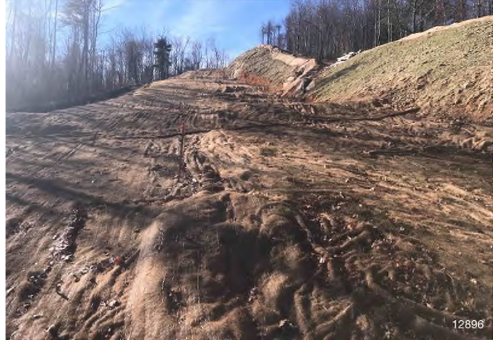
Figure 4: STA 12881+00 – Controls in place and functioning properly. Area stabilized with straw. BRG: 45°NE (T) LAT: 37.148881 LON: -80.119800 ±10121ft ALT: 2659ft
