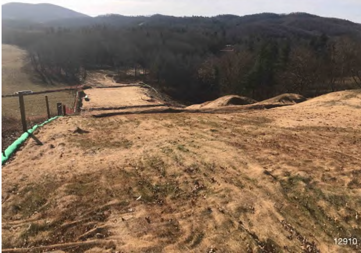
Figure 3: STA 12892+00 – Controls in place and functioning properly. Area stabilized with straw. BRG: 220°SW (T) LAT: 37.149909 LON: -80.133341 ±328ft ALT: 2737ft
