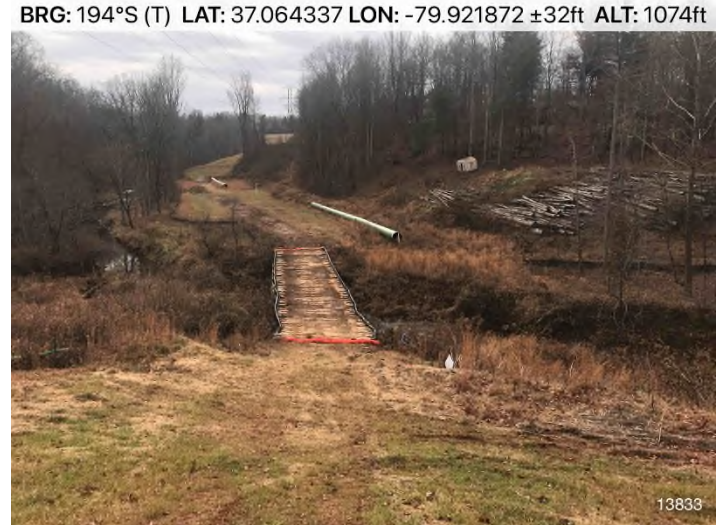
Figure 4: STA 13784+00 – Controls in place and functioning properly. Area stabilized with straw. BRG: 287°W (T) LAT: 37.069237 LON: -79.946694 ±9051ft ALT: 1062ft
