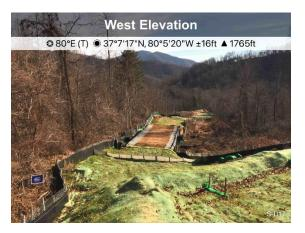
Figure 2: St13116 ESC crews were actively temporarily stabilizing with matting.
