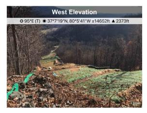
Figure 4: St 13141+07 ECD's have been installed.
