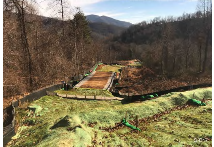
Figure 2: Stream S-D17 – Controls in place and functioning properly. BRG: 94°E (T) LAT: 37.121680 LON: -80.088925 ±32ft ALT: 1792ft
