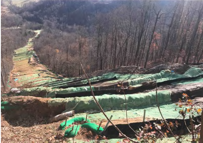
Figure 1: STA 13121+00 – Controls in place and functioning properly. Area stabilized with erosion matting. BRG: 123°SE (T) LAT: 37.121969 LON: -80.094099 ±32ft ALT: 2410ft
