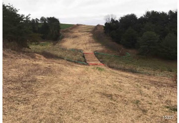
Figure 2: STA 15327+00 – Controls in place and functioning properly. Area stabilized with straw. BRG: 121°SE (T) LAT: 36.928286 LON: -79.522008 ±32ft ALT: 707ft
