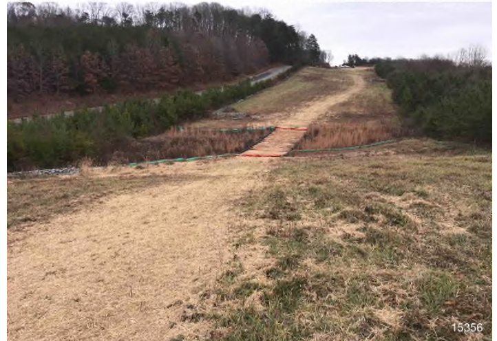
Figure 4: STA 15356+00 – Controls in place and functioning properly. Area stabilized with straw BRG: 97°E (T) LAT: 36.923368 LON: -79.514165 ±16ft ALT: 740ft
