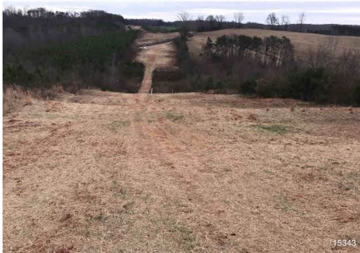
Figure 3: STA 15343+00 – Controls in place and functioning properly. Area stabilized with straw BRG: 126°SE (T) LAT: 36.918542 LON: -79.531105 ±9708ft ALT: 752ft
