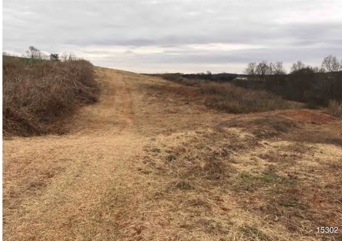
Figure 1: STA 15302+00 – Controls in place and functioning properly. Area stabilized with straw BRG: 149°SE (T) LAT: 36.931038 LON: -79.531548 ±213ft ALT: 774ft
