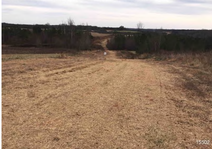
Figure 1: STA 15502+00 – Controls in place and functioning properly. Area stabilized with straw BRG: 97°E (T) LAT: 36.913131 LON: -79.468459 ±11742ft ALT: 918ft
