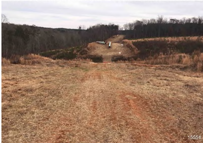
Figure 3: STA 15554+00 – Controls in place and functioning properly. Area stabilized with straw BRG: 98°E (T) LAT: 36.894303 LON: -79.407332 ±12604ft ALT: 789ft
