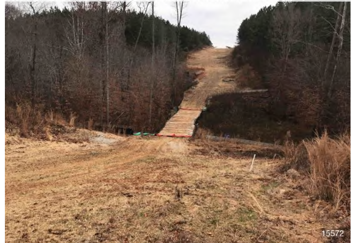
Figure 4: STA 15572+00 – Controls in place and functioning properly. Area stabilized with straw BRG: 98°E (T) LAT: 36.898317 LON: -79.450577 ±16420ft ALT: 849ft
