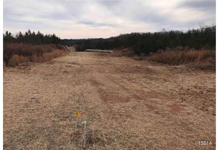
Figure 2: STA 15514+00 – Controls in place and functioning properly. Area stabilized with straw. BRG: 88°E (T) LAT: 36.904874 LON: -79.470921 ±8415ft ALT: 843ft
