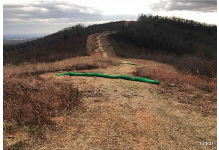
Figure 4: STA 13440+00 – Controls in place and functioning properly. BRG: 136°SE (T) LAT: 37.090219 LON: -80.019881 ±16ft ALT: 1707ft
