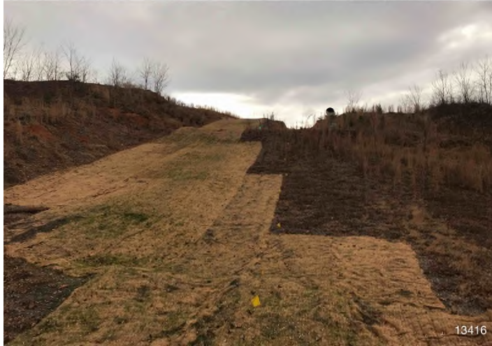
Figure 1: STA 13416+00 – Controls in place and functioning properly. Area stabilized with erosion matting. BRG: 107°E (T) LAT: 37.092180 LON: -80.027055 ±16ft ALT: 1493ft
