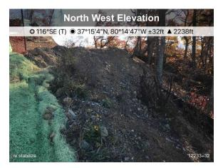
Figure 2: St12205 area requires re stabilization.
