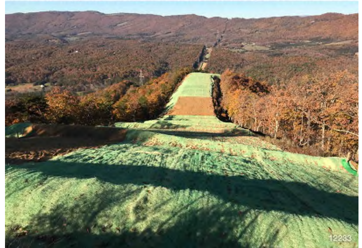
Figure 4: STA 12233+00 – Controls in place and functioning properly. Area stabilized erosion matting.
