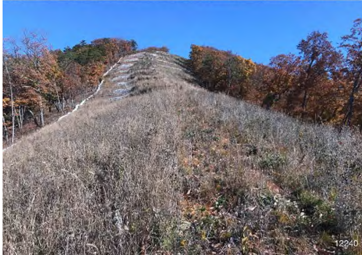
Figure 3: STA 12209+00 – Controls in place and functioning properly. Area stabilized erosion matting.
