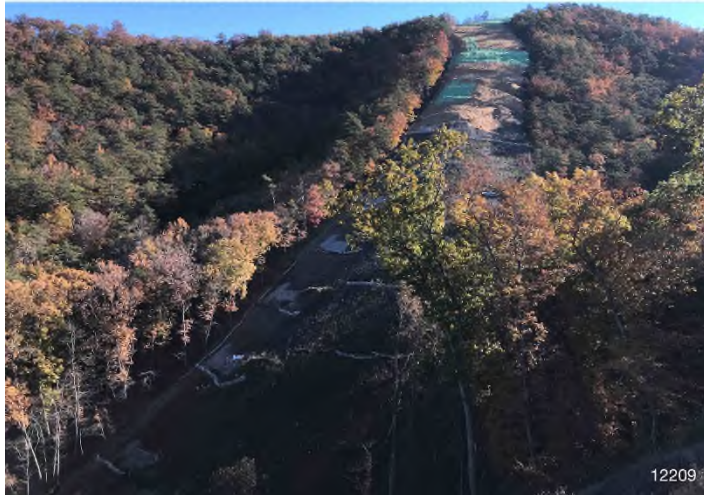
Figure 3: STA 12209+00 – Controls in place and functioning properly. Area stabilized erosion matting.
