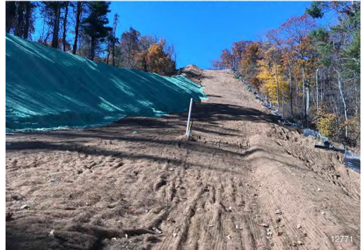
Figure 4: STA 12771+00 – Controls in place and functioning properly. Area stabilized erosion matting.
