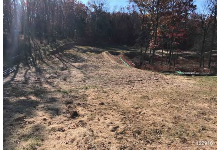
Figure 4: STA 12771+00 – Controls in place and functioning properly. Area stabilized erosion matting.
