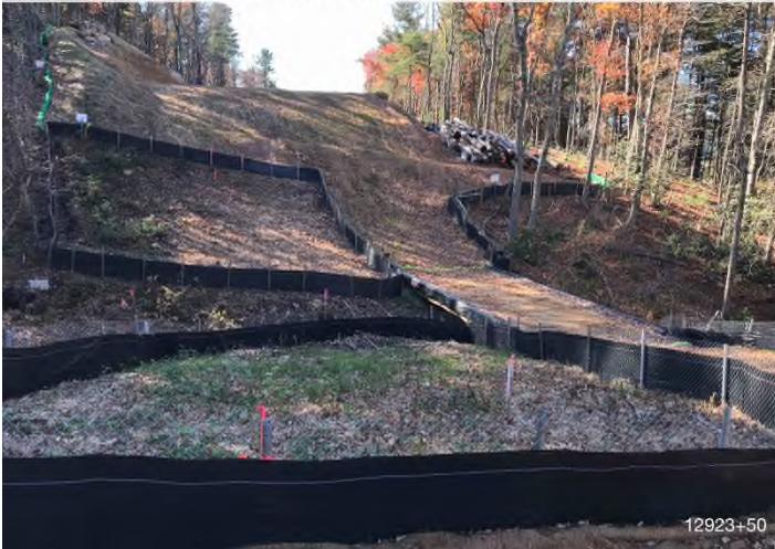
Figure 3: STA 12923+50 – Controls in place and functioning properly. Area stabilized erosion matting.
