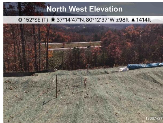
Figure 4: St 12367+27 ECD's are in place.
