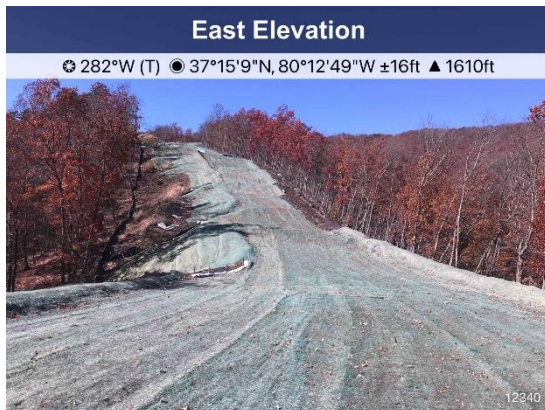
Figure 3: St 12340 ECD's are in place.
