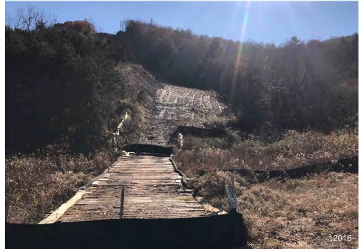
Figure 4: STA 12016+00 – Controls in place and functioning properly. Area stabilized erosion matting. BRG: 148°SE (T) LAT: 37.267227 LON: -80.313112 ±16ft ALT: 1649ft
