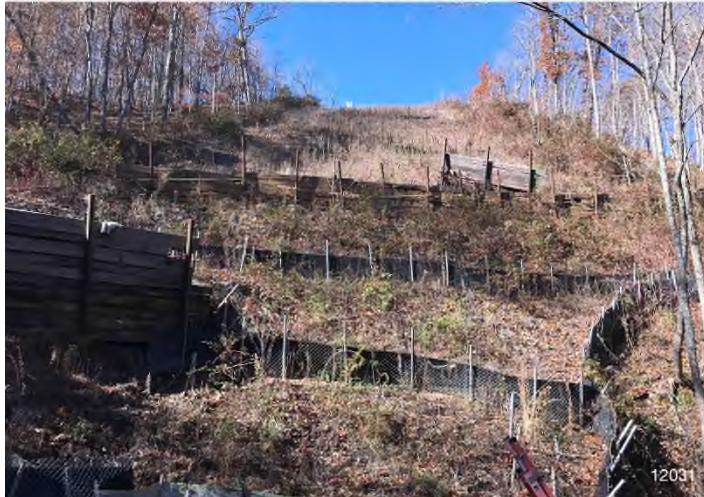
Figure 3: STA 12031+00 – Controls in place and functioning properly. Area stabilized erosion matting. BRG: 292°W (T) LAT: 37.265060 LON: -80.308525 ±32ft ALT: 1735ft
