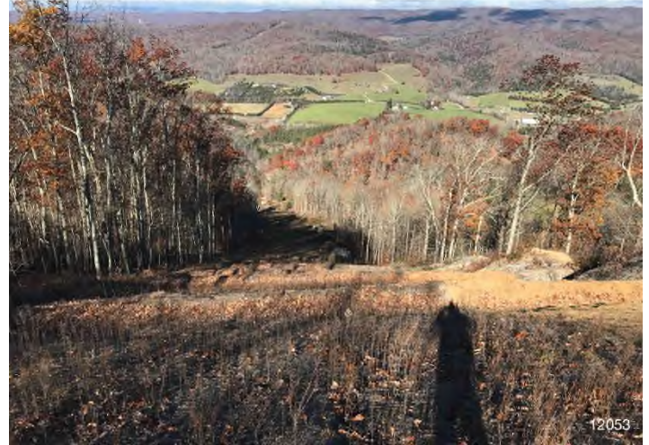
Figure 2: STA 12053+00 – Controls in place and functioning properly. Area stabilized erosion matting. BRG: 336°NW (T) LAT: 37.271777 LON: -80.313685 ±921ft ALT: 1679ft
