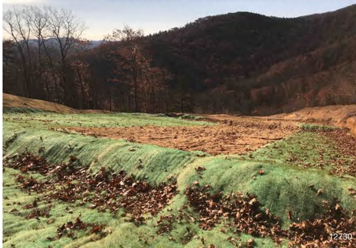
Figure 3: STA 12755+00 – Controls in place and functioning properly. Area stabilized erosion matting. BRG: 93°E (T) LAT: 37.180673 LON: -80.134236 ±22913ft ALT: 3068ft
