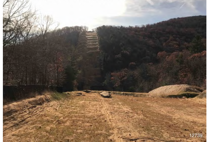
Figure 4: STA 12765+00 – Controls in place and functioning properly. Area stabilized erosion matting. BRG: 73°E (T) LAT: 37.179265 LON: -80.145367 ±98ft ALT: 3091ft
