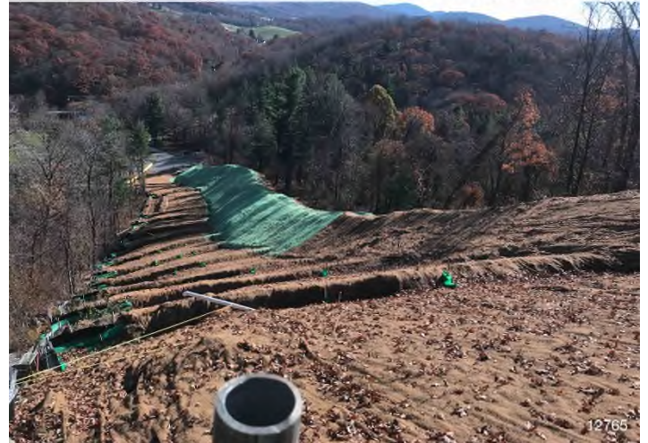
Figure 4: STA 12765+00 – Controls in place and functioning properly. Area stabilized erosion matting. BRG: 73°E (T) LAT: 37.179265 LON: -80.145367 ±98ft ALT: 3091ft
