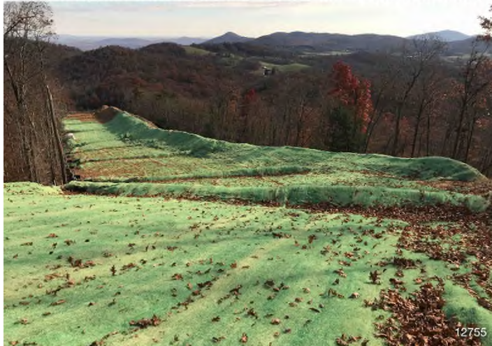
Figure 3: STA 12755+00 – Controls in place and functioning properly. Area stabilized erosion matting. BRG: 93°E (T) LAT: 37.180673 LON: -80.134236 ±22913ft ALT: 3068ft
