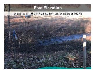
Figure 2: St13203 area has been temporarily stabilized with matting.
