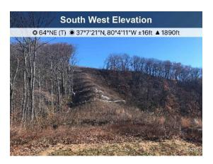
Figure 4: Completed crossing S-II4, ECD's are in place.
