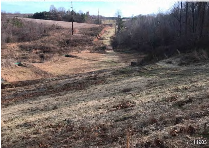
Figure 3: STA 14903+00 – Controls in place and functioning properly.
