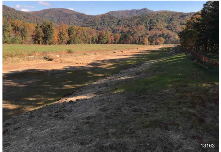
Figure 4: STA 13163+00 – Controls in place and functioning properly. Area stabilized with straw.
