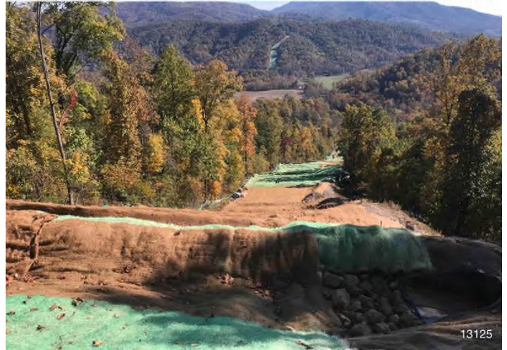
Figure 4: STA 13163+00 – Controls in place and functioning properly. Area stabilized with straw.
