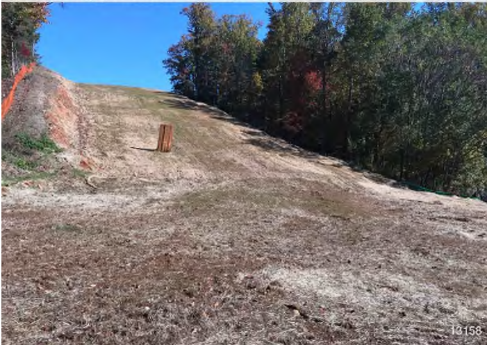
Figure 3: STA 13158+00 – Controls in place and functioning properly. Area stabilized with straw.
