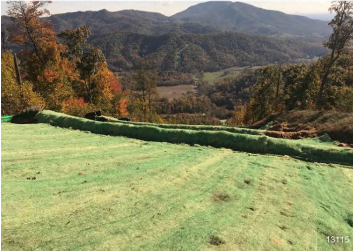
Figure 3: STA 13158+00 – Controls in place and functioning properly. Area stabilized with straw.
