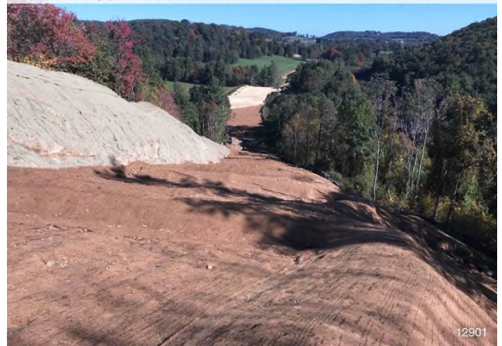
Figure 4: STA 12901+00 – Controls in place and functioning properly. Area stabilized with erosion matting. BRG: 30°NE (T) LAT: 37.145966 LON: -80.137374 ±17060ft ALT: 2831ft
