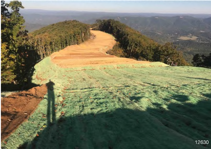
Figure 1: STA 12630+00 – Controls in place and functioning properly. Area stabilized with erosion matting and straw. BRG: 323°NW (T) LAT: 37.193329 LON: -80.175997 ±164ft ALT: 3048ft
