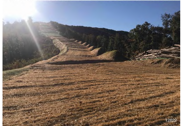
Figure 2: STA 12622+00 – Controls in place and functioning properly. Area stabilized with straw. BRG: 151°SE (T) LAT: 37.195210 LON: -80.178369 ±98ft ALT: 3432ft
