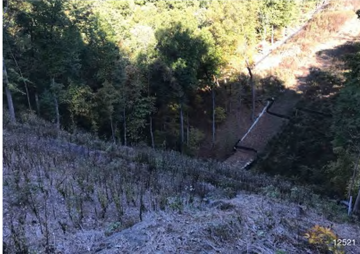
Figure 3: STA 12490+00 – Controls in place and functioning properly. Area being re-stabilized with erosion matting.
