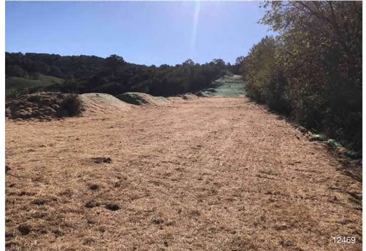
Figure 4: STA 12469+00 – Controls in place and functioning properly. Area stabilized with erosion matting and straw.
