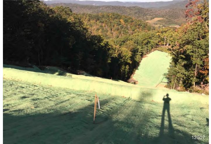
Figure 4: STA 12469+00 – Controls in place and functioning properly. Area stabilized with erosion matting and straw.
