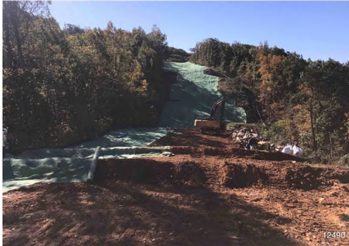
Figure 3: STA 12490+00 – Controls in place and functioning properly. Area being re-stabilized with erosion matting.
