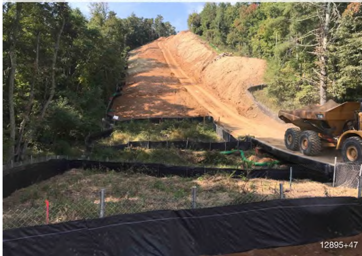
Figure 3: STA 12895+47 – Controls in place and functioning properly.
