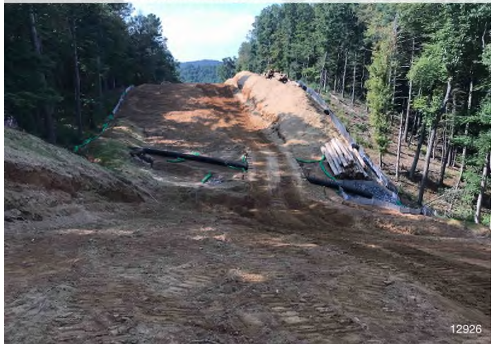
Figure 4: STA 12926+00 – Controls in place and functioning properly.
