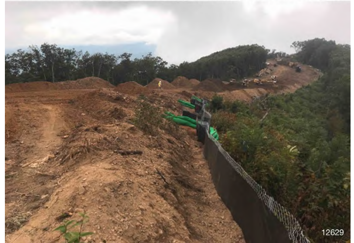
Figure 4: STA 12629+00 – Controls in place and functioning properly.
