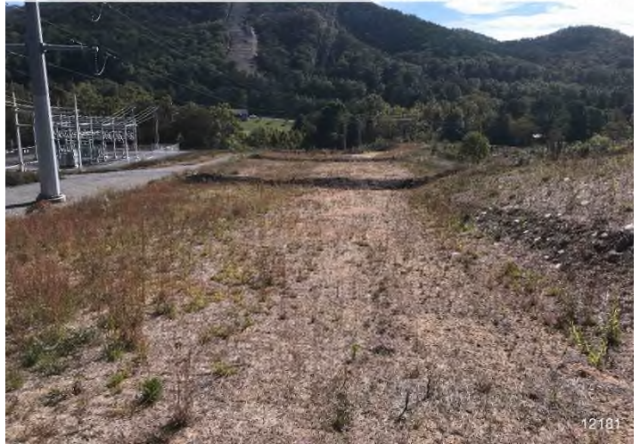
Figure 4: ATWS 1446 – Controls in place and functioning properly. Area stabilized with straw.
