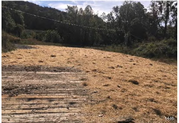
Figure 4: ATWS 1446 – Controls in place and functioning properly. Area stabilized with straw.
