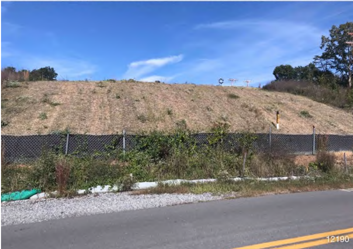
Figure 3: STA 12190+00 – Controls in place and functioning properly at Bradshaw Road crossing.
