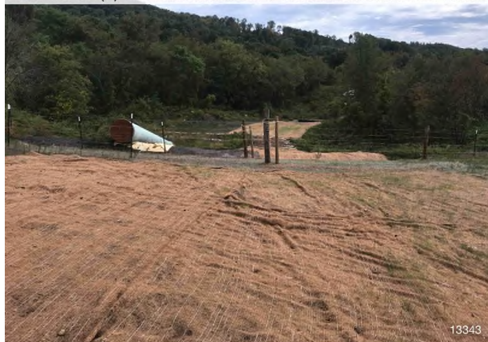
Figure 1: STA 13343+00 – Controls in place and functioning properly. Area stabilized with erosion matting. BRG: 116°SE (T) LAT: 37.103922 LON: -80.043198 ±16ft ALT: 1568ft
