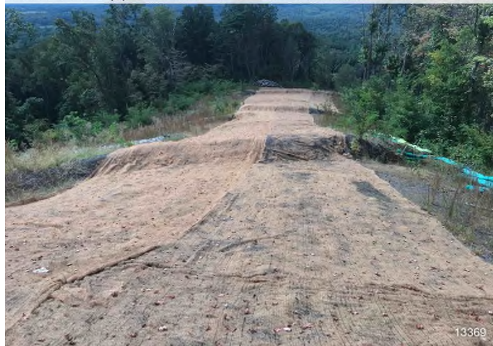
Figure 3: STA 13369+00 – Controls in place and functioning properly. Area stabilized with erosion matting. BRG: 232°SW (T) LAT: 37.101381 LON: -80.036380 ±16ft ALT: 1744ft
