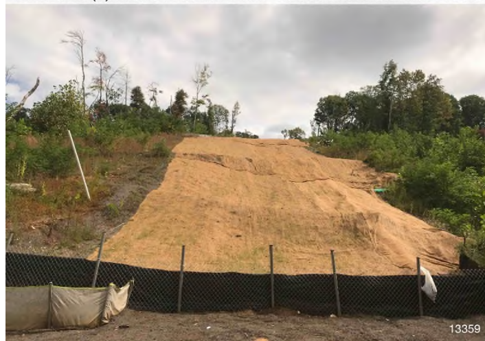
Figure 2: STA 13359+00 – Controls in place and functioning properly. Area stabilized with erosion matting. BRG: 87°E (T) LAT: 37.100967 LON: -80.039578 ±16ft ALT: 1480ft
