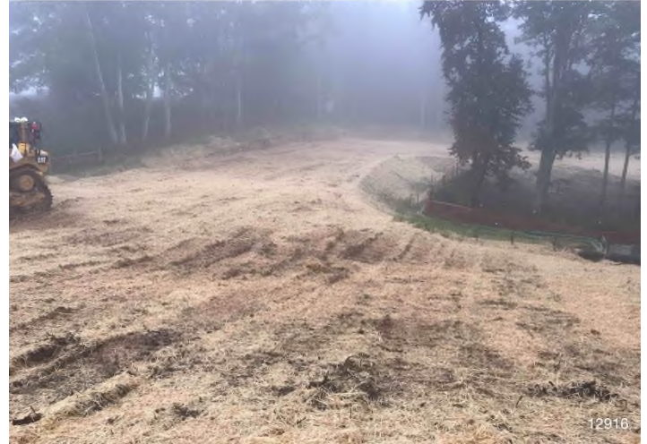
Figure 2: STA 12916+00 – Controls in place and functioning properly. Area stabilized with straw. BRG: 148°SE (T) LAT: 37.144511 LON: -80.137618 ±16ft ALT: 2689ft
