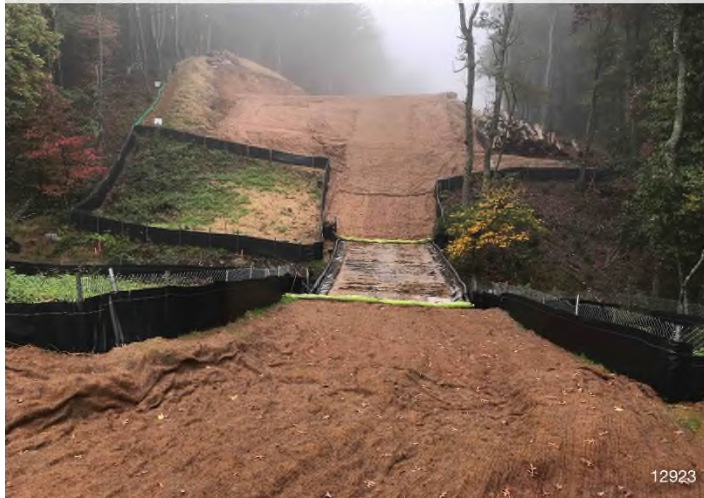
Figure 3: STA 12923+00 – Controls in place and functioning properly. Area stabilized with erosion matting. BRG: 188°S (T) LAT: 37.143462 LON: -80.138072 ±3776ft ALT: 2676ft
