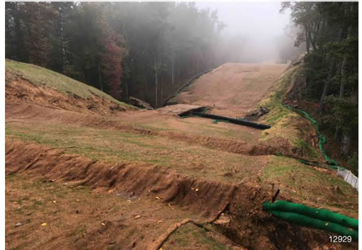
Figure 4: STA 12929+00 – Controls in place and functioning properly. Area stabilized with erosion matting. BRG: 2°N (T) LAT: 37.141357 LON: -80.138884 ±32ft ALT: 2681ft
