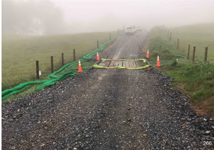
Figure 1: MVP-RO-286 – Controls in place and functioning properly along access road. BRG: 267°W (T) LAT: 37.144853 LON: -80.135831 ±16ft ALT: 2697ft
