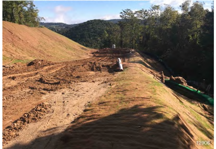
Figure 4: STA 12871+00 – Controls in place and functioning properly. Area stabilized with straw.
