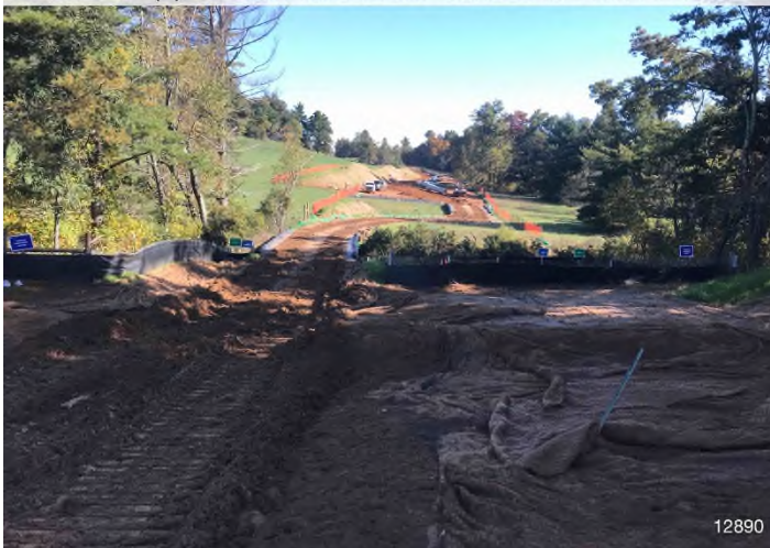
Figure 3: STA 12890+00 – Controls in place and functioning properly. Area stabilized with erosion matting.
