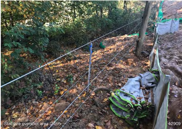
Figure 3: STA 12890+00 – Controls in place and functioning properly. Area stabilized with erosion matting.
