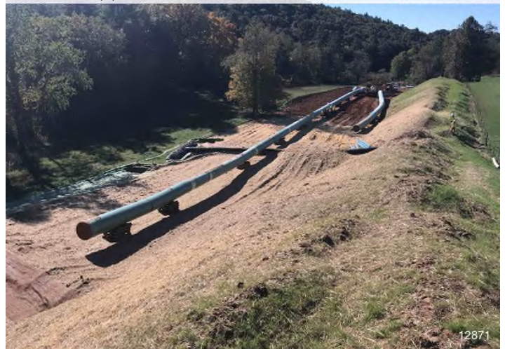
Figure 4: STA 12871+00 – Controls in place and functioning properly. Area stabilized with straw.
