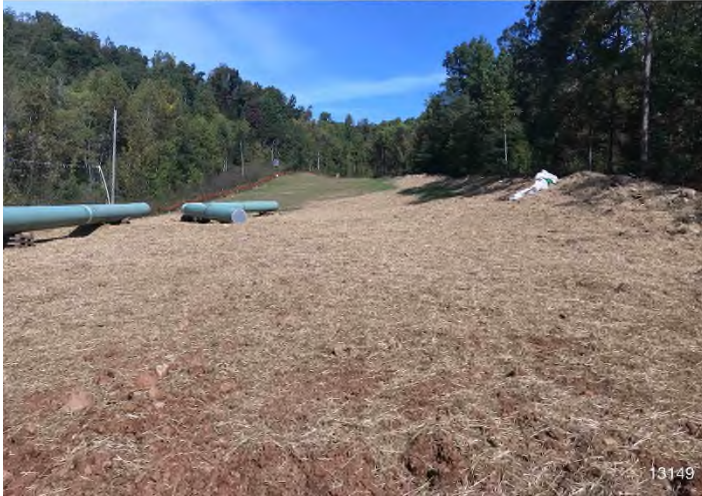
Figure 3: STA 13163+00 – Controls in place and functioning properly. Area stabilized with straw.
