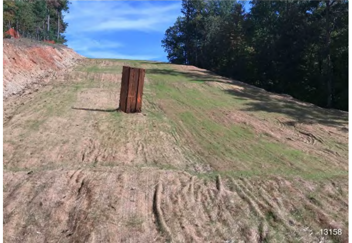
Figure 4: STA 13186+00 – Controls in place and functioning properly. Area stabilized with erosion matting.
