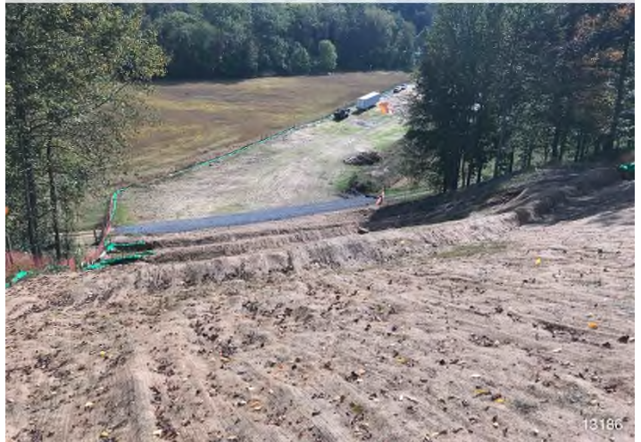
Figure 4: STA 13186+00 – Controls in place and functioning properly. Area stabilized with erosion matting.
