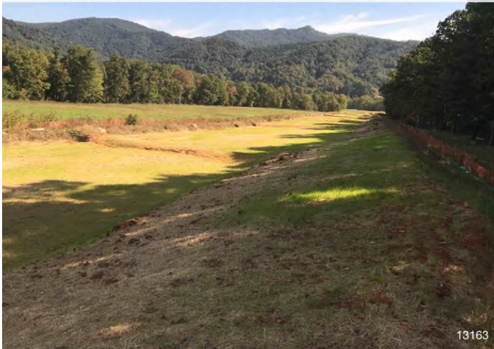
Figure 3: STA 13163+00 – Controls in place and functioning properly. Area stabilized with straw.
