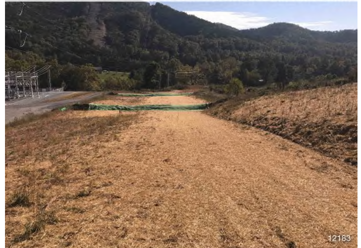
Figure 4: STA 12183+00 – Controls in place and functioning properly. Area stabilized with straw. BRG: 101°E (T) LAT: 37.252721 LON: -80.261836 ±16ft ALT: 1366ft
