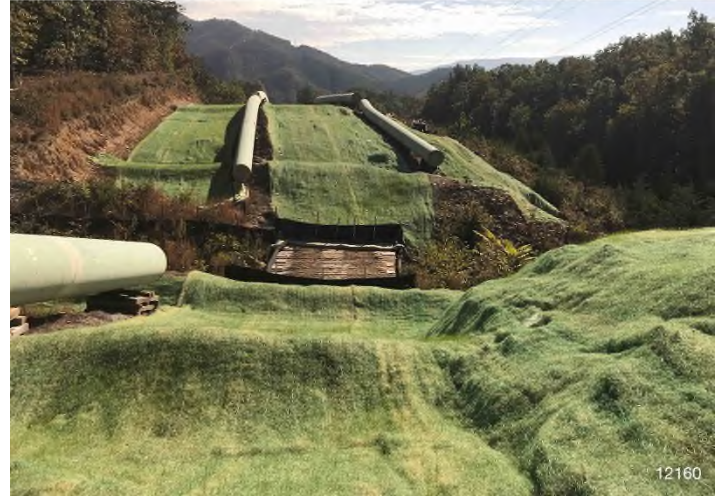
Figure 2: STA 12160+00 – Controls in place and functioning properly. Area stabilized with erosion matting. BRG: 112°E (T) LAT: 37.237022 LON: -80.260660 ±6463ft ALT: 1553ft
