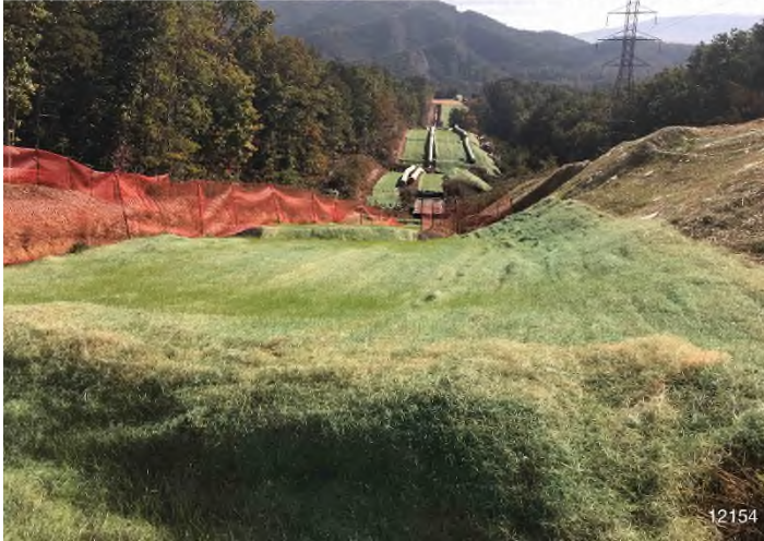
Figure 1: STA 12154+00 – Controls in place and functioning properly. Area stabilized with erosion matting. BRG: 96°E (T) LAT: 37.254865 LON: -80.271101 ±32ft ALT: 1542ft
