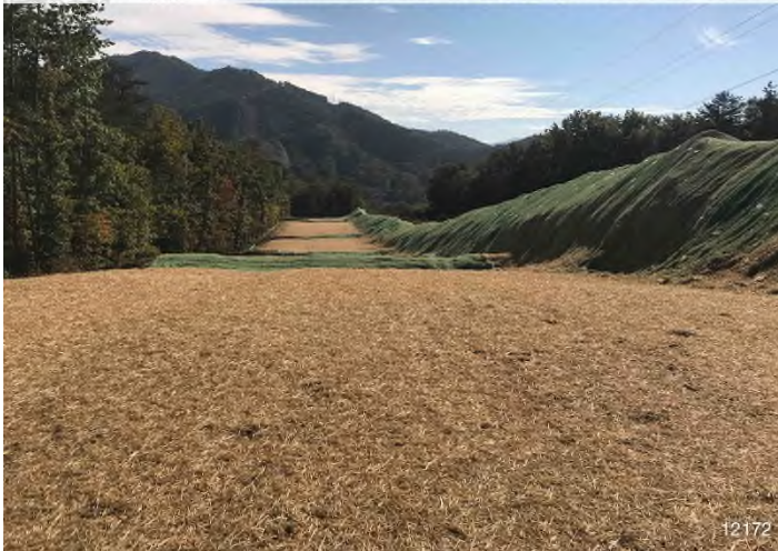
Figure 3: STA 12172+00 – Controls in place and functioning properly. Area stabilized with straw. BRG: 104°E (T) LAT: 37.253976 LON: -80.265243 ±32ft ALT: 1423ft
