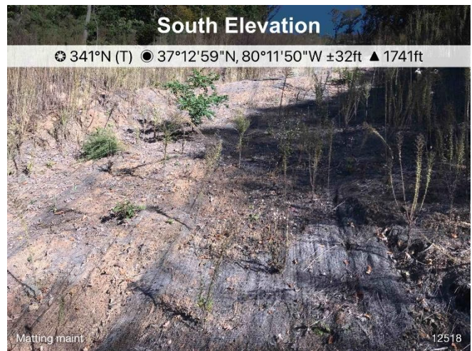
Figure 4: St 12518 ROW requires additional stabilization
