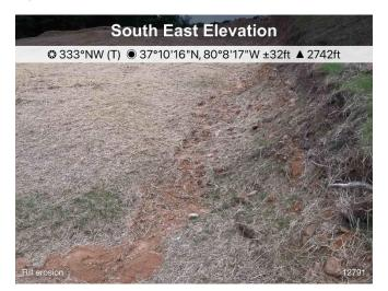
Figure 3: St 12789 fill slope lacks stabilization
