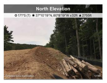
Figure 4: St 12776+80-12777+20 rill erosion requires repair
