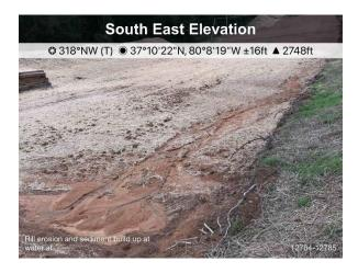
Figure 2:St 12791 rill erosion requires repair
