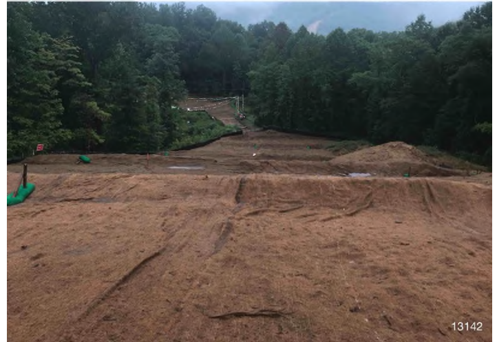
Figure 4: Stream S-EF55 – Controls in place and functioning properly. Area stabilized with erosion matting.
