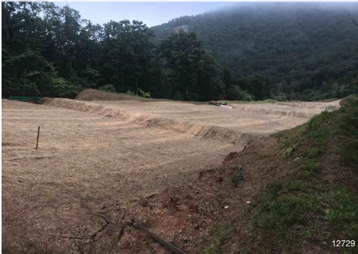
Figure 3: STA 12729+00 – Controls in place and functioning properly. Area stabilized with erosion matting.
