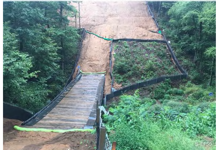
Figure 4: Stream S-EF55 – Controls in place and functioning properly. Area stabilized with erosion matting.
