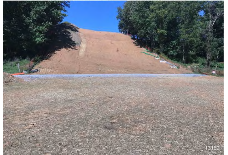
Figure 4: STA 12126+00 – Controls in place and functioning properly. Area stabilized with straw..
