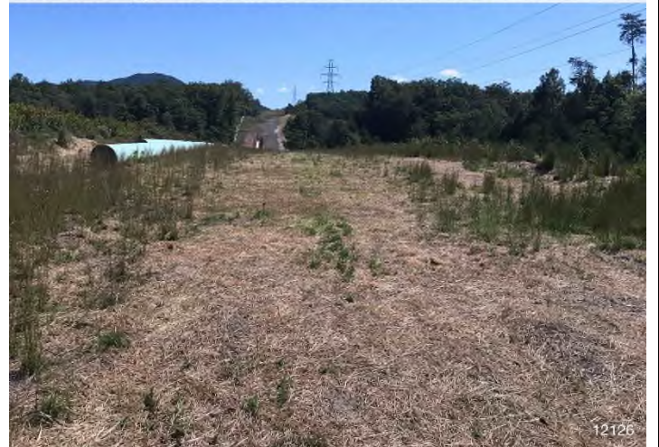
Figure 4: STA 12126+00 – Controls in place and functioning properly. Area stabilized with straw..
