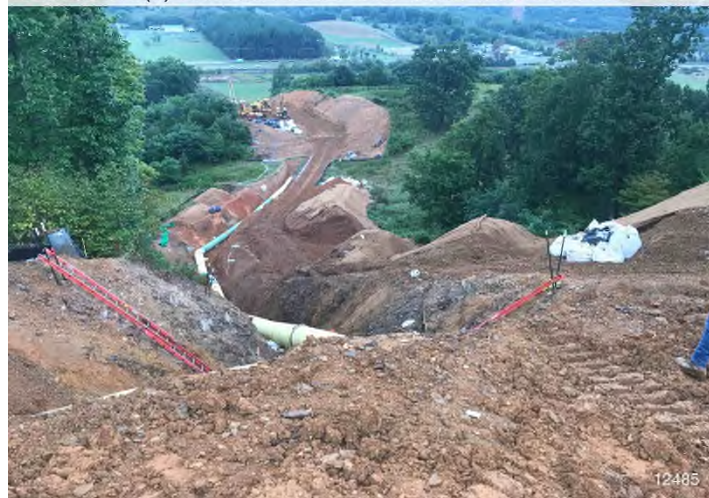
Figure 2: STA 12480+00 – Controls in place and functioning properly.
