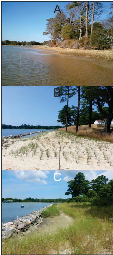
Figure 4-2-6. Photos of reach 3 at Occohannock on the Bay A), before construction (March 2013), B) after construction (March 2013), C) after planting (May 2013), C) after 5 years.
