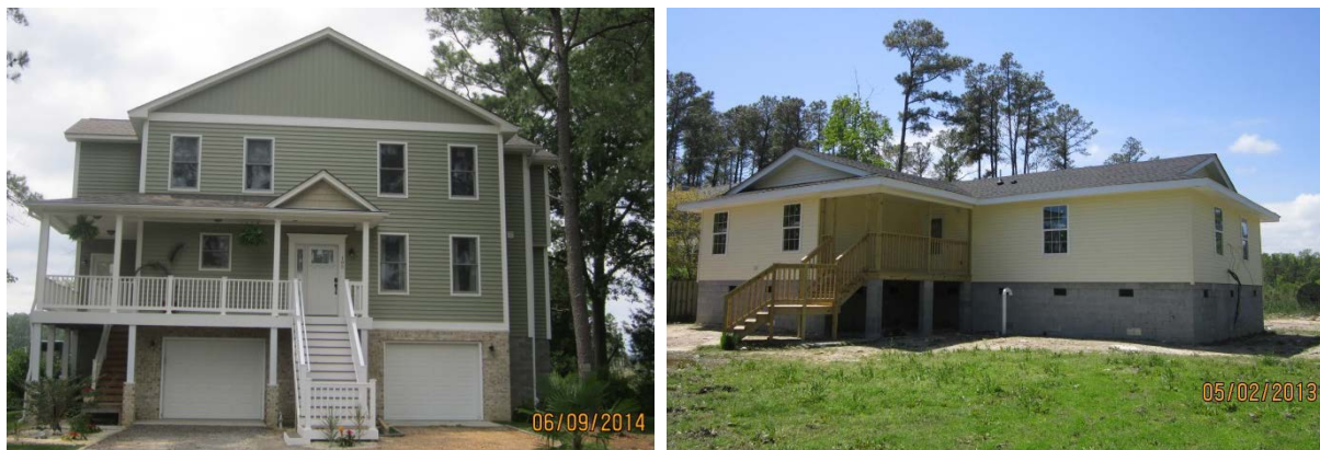
Figure 15: House with foundation type coded as “GAR/U” (left) and house with foundation type coded as “ELEV” (right). Images obtained from York County Property Information portal https://maps.yorkcounty.gov/York/Account/Login
