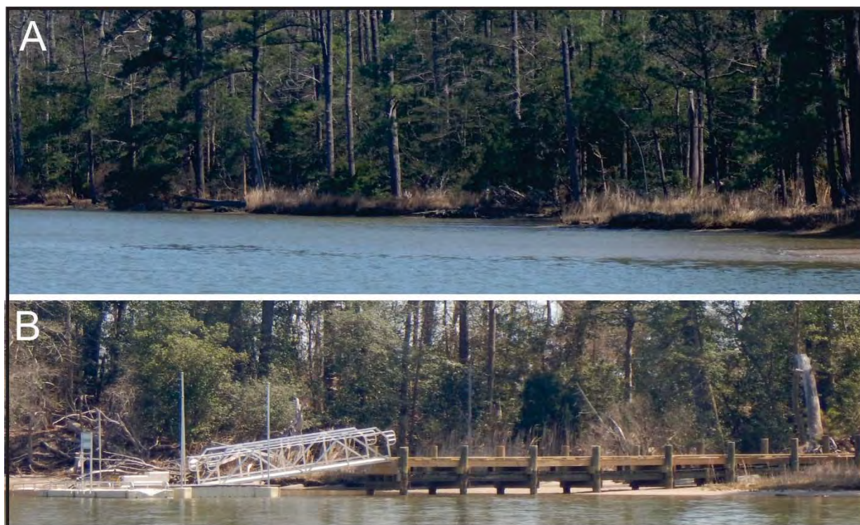
Figure 4-10. A) Low, undercut upland banks with intermittent eroding marsh fringes occur along much of Reach 1 along Mulberry Creek. B) An access pier along Reach 1.
