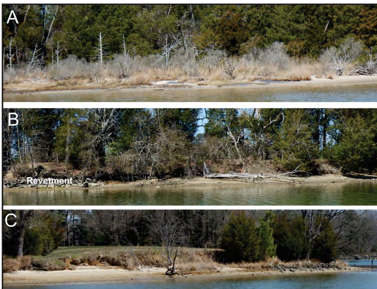
Figure 4-12. A) Reach IIIA shoreline is a low eroding marsh fringe on sandy spit. B) Eroding upland adjacent to boat ramp. Note existing rock for shore erosion control. C) Eroding point at Bel Air Guest House on Deep Creek.
