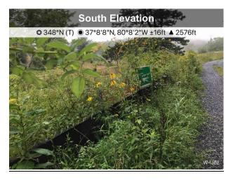
Figure 4: Designated crossing S-Z16, ECD's are in place.
