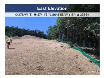
Figure 2: St12720 temporary waterbars in place and stockpiles have been stabilized.
