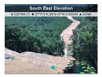
Figure 3: Designated crossing S-EF34B, ECD's are in place.
