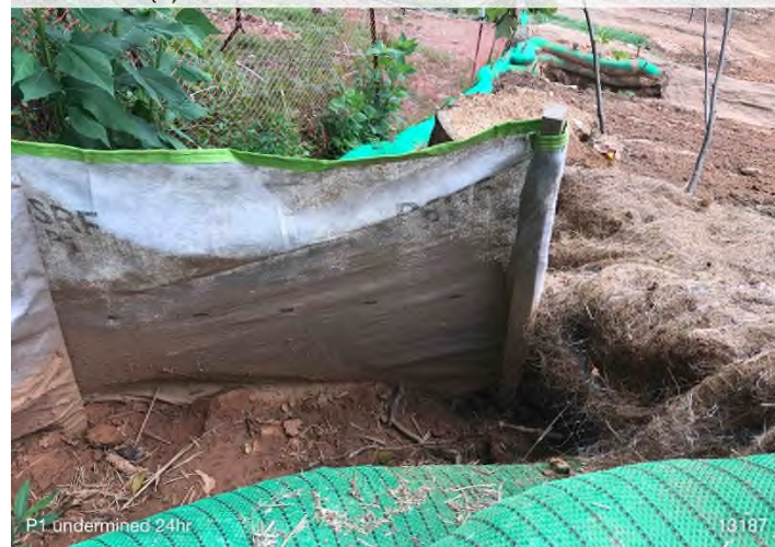
Figure 4: STA 13187+00 – P1 undermined.
