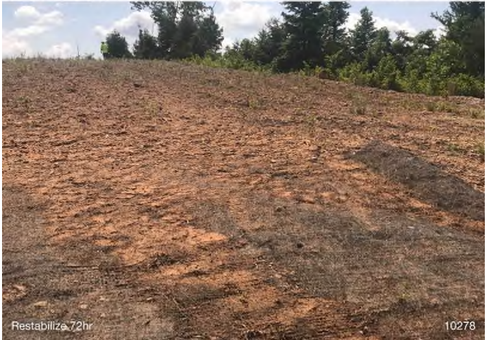
Figure 4: STA 12098+40 to 12100+00 – Re-stabilization needed.
