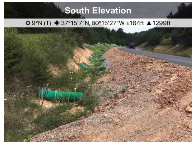
Figure 4: Construction road site not associated with the MVP project, fill slope and ditch line not adequately stabilized near S-C21.
