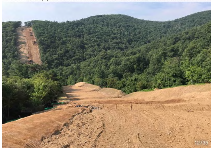
Figure 3: STA 12742+00 – Controls in place and functioning properly.
