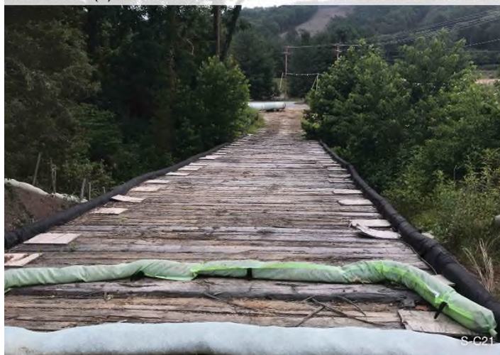
Figure 4: Stream S-C21 – Controls in place and functioning properly along Bradshaw Creek.
