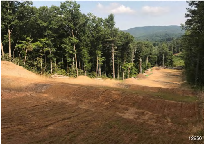
Figure 3: STA 12950+00 – Controls in place and functioning properly. Area stabilized with straw and erosion control matting. BRG: 318°NW (T) LAT: 37.136478 LON: -80.138581 ±32ft ALT: 2726ft
