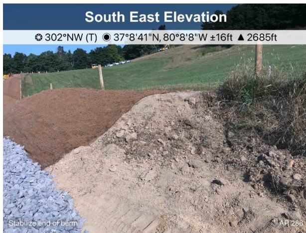
Figure 3: AR 286 end of berm lacks stabilization
