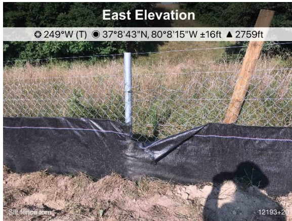
Figure 1: St 12913+20 SSF torn
