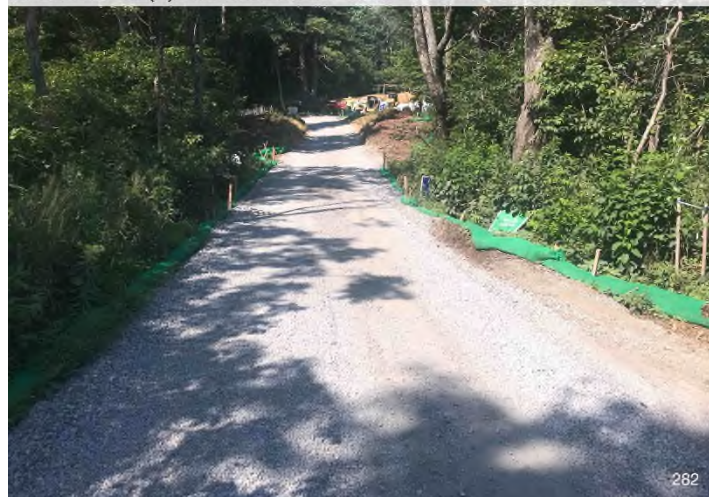
Figure 4: Stream S-EF33 – Controls in place and functioning properly along stream crossing.
